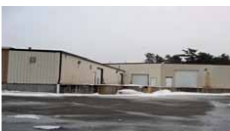
PLYMOUTH Industrial - Warehouse 41,500 SF - $1,700,000
