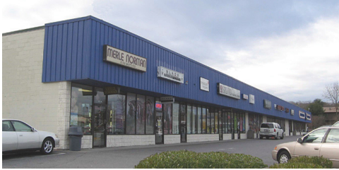
331 State Road Plaza - North Dartmouth, MA
